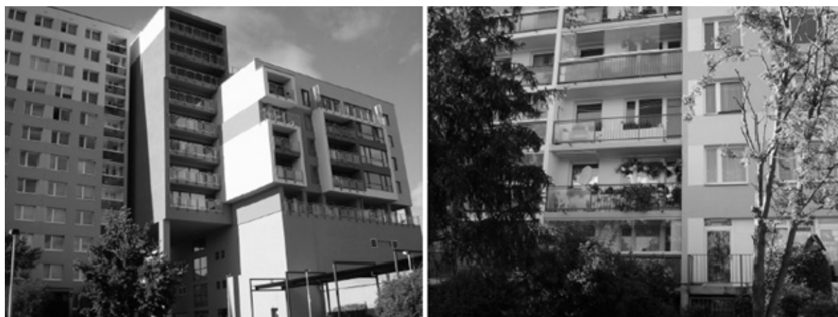
Figure 5: New apartment building and regenerated panel house in Jižní Město
